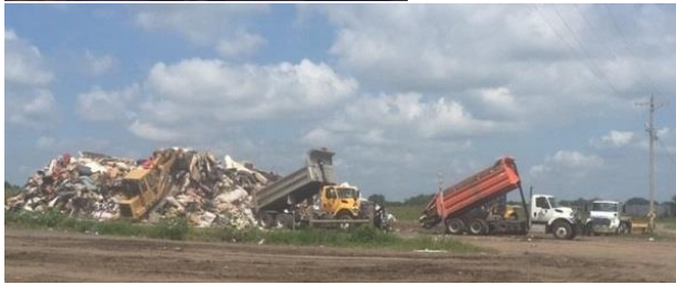
(Top) Flood Debris cleanup – sometimes it takes super heroes. (Bottom) Both the City of Des Moines & City of West Des Moines staff helping with debris. removal.
